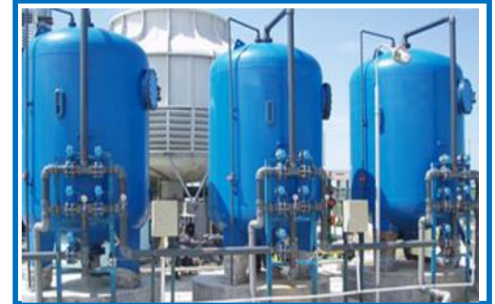
De - Mineralization Plant
