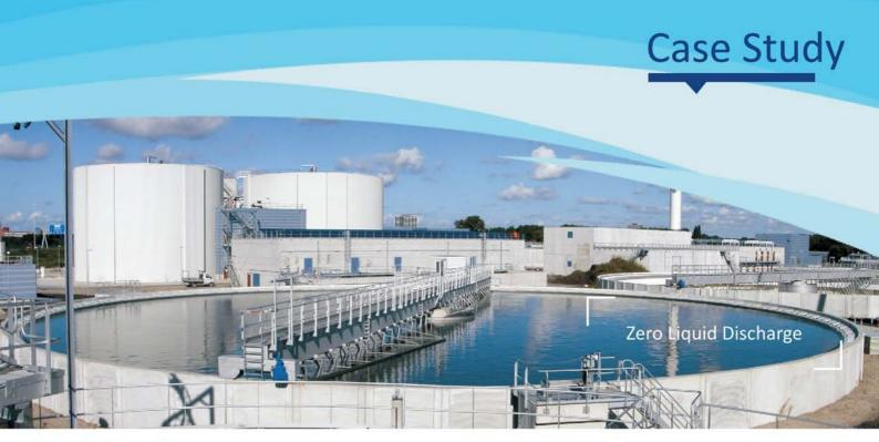
Introduction | Sparkle Clean Tech Pvt Ltd. has designed, supplied, commissioned 400 KLD Effluent Treatment using Membrane Bio Reactor and Reverse Osmosis process for a malt processing industry.
